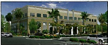
Newport National Corp. is developing Nordahl Medical Centre, a 55,450-square-foot medical condominium building in San Marcos, Calif.
